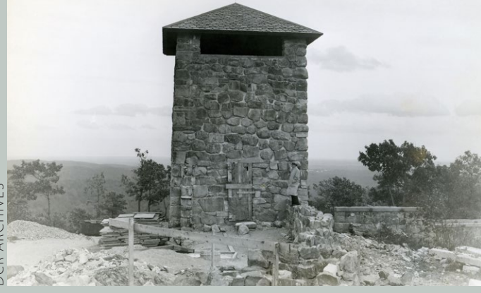
ELIOT TOWER CONSTRUCTION, 1937
